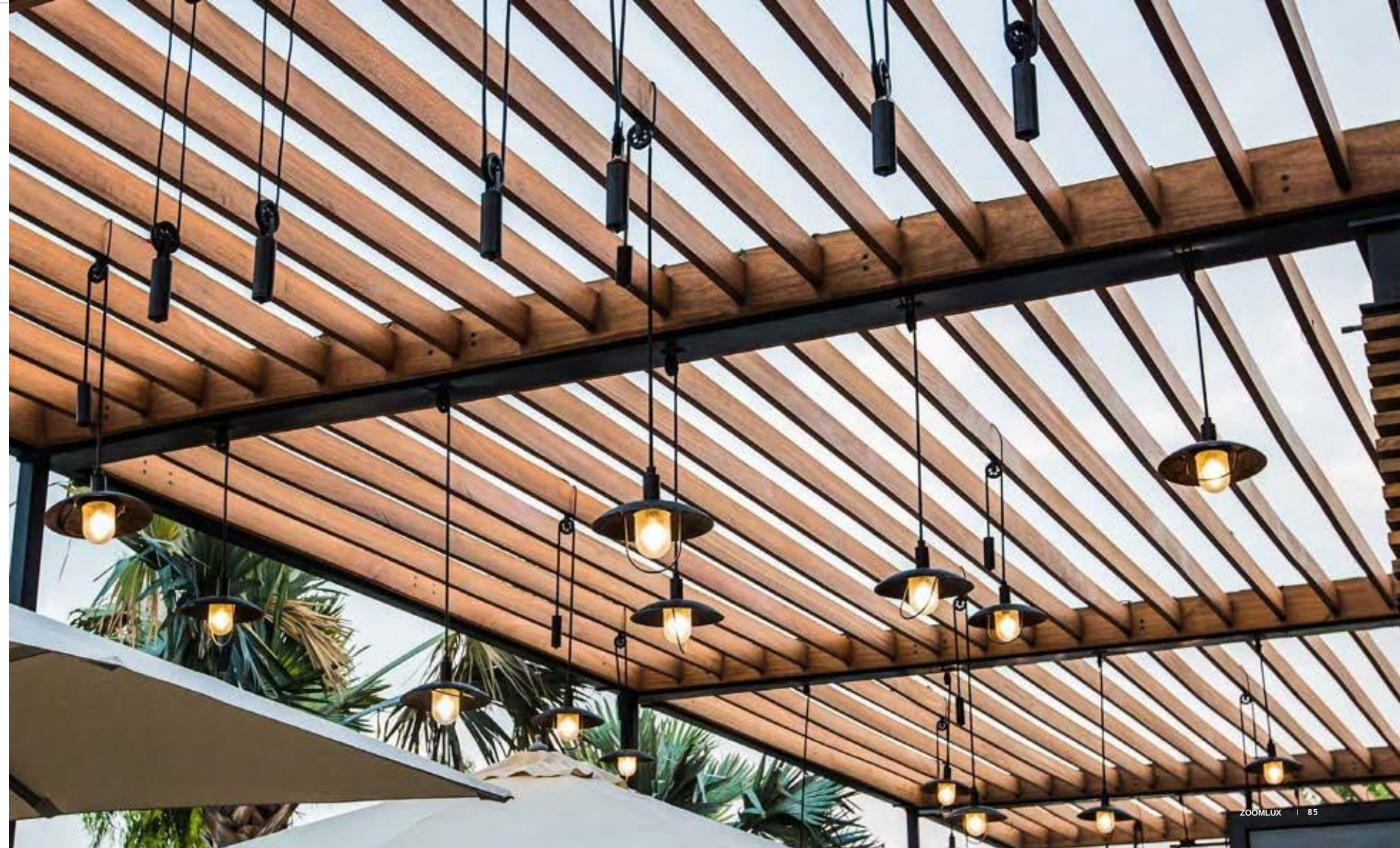
SS Rod used to give the effect of a weight and pulley system while keeping the luminaire safely fixed in place
